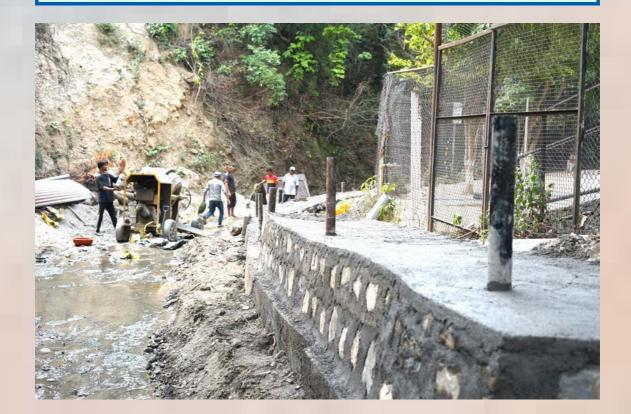
The embankment that supports the sports field suffers from continuous erosion from the adjacent stream. Over time pieces of this reinforcement have been washed away, due to which a cavity had been created under the sports field. To rectify the problem, gaps were filled with rock and concrete, and a new solid wall was built alongside to prevent the flow of water from eroding the base of the sports field.
